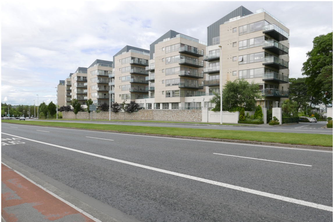
Figure 12.7 - Seven storey apartment blocks at Beechwood Court at Galloping Green on the N11 National Primary Route.
