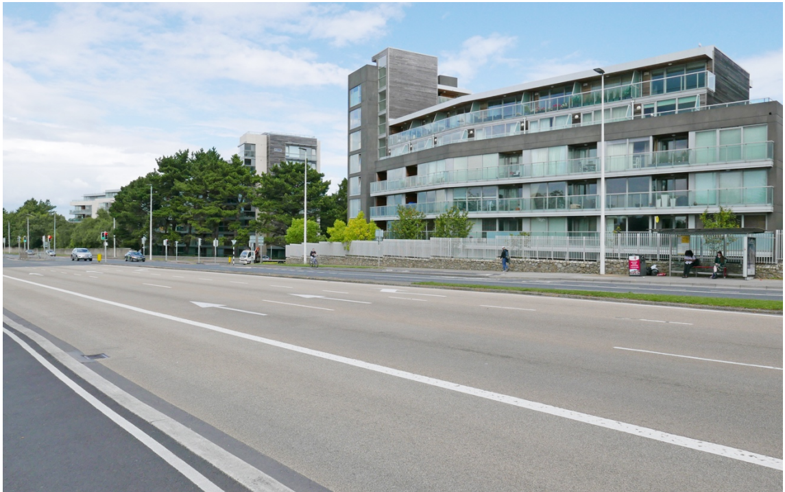
Figure 12.8 - The six to eight storey Thornwood Apartments (left) and the five to seven storey Booterstown Wood apartments (right) at the junction of Booterstown Avenue with the N11 National Primary Route.
